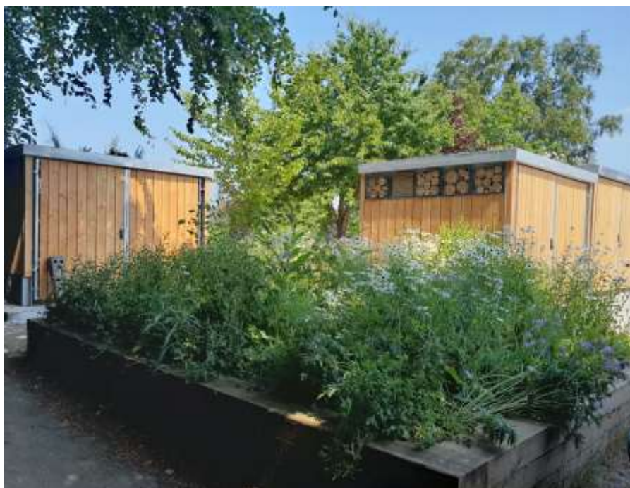
Figure 11. Green Roof Bin Shelters at Gnoll Country Park
